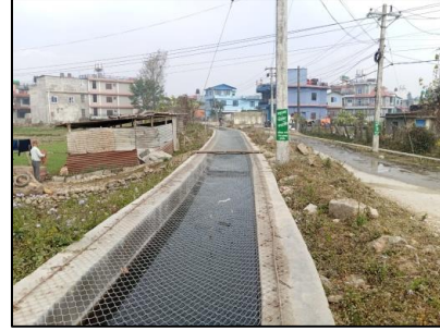
Figure 10: Headrace canal
