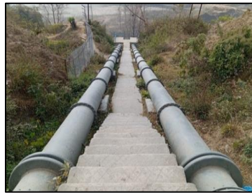
Figure 13: Penstock pipes
