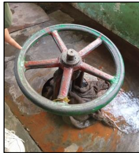
Figure 15: Main Inlet Valve
