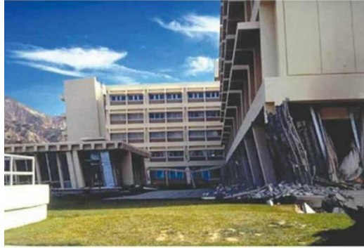
Figure 2 : Soft-Storey failure of Olive View Hospital during 1971
